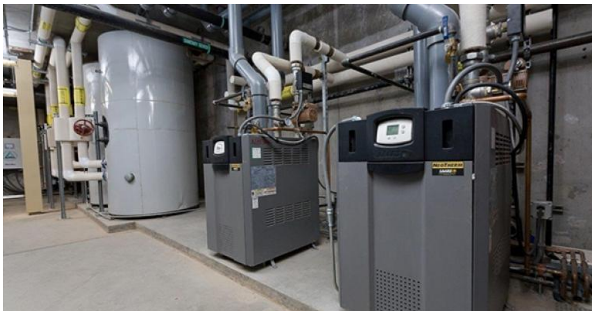
Domestic hot water plant of a health center
