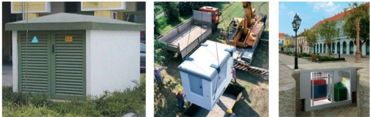
Transformer stations outside the building (above ground and underground)
