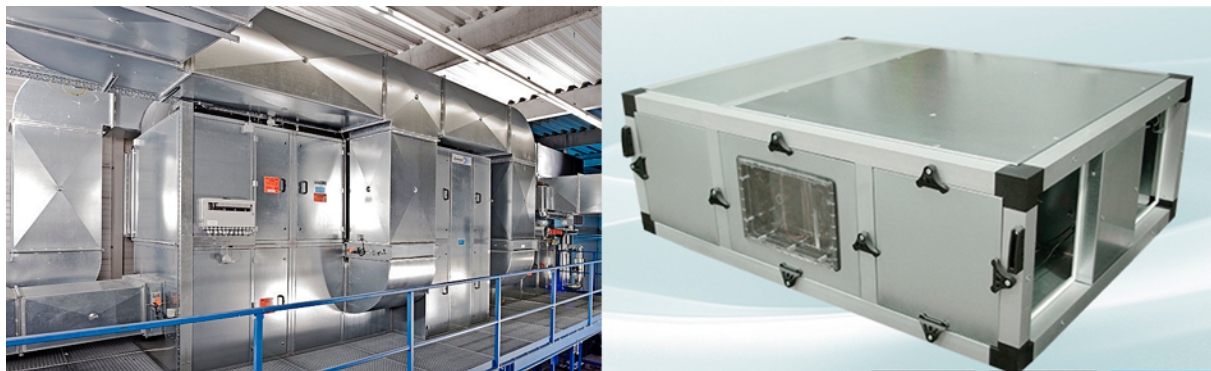
Ventilation plant and compact ventilation unit with heat-exchanger
