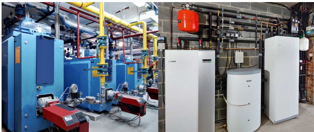
Gas boiler plant and domestic boiler with heat pump
