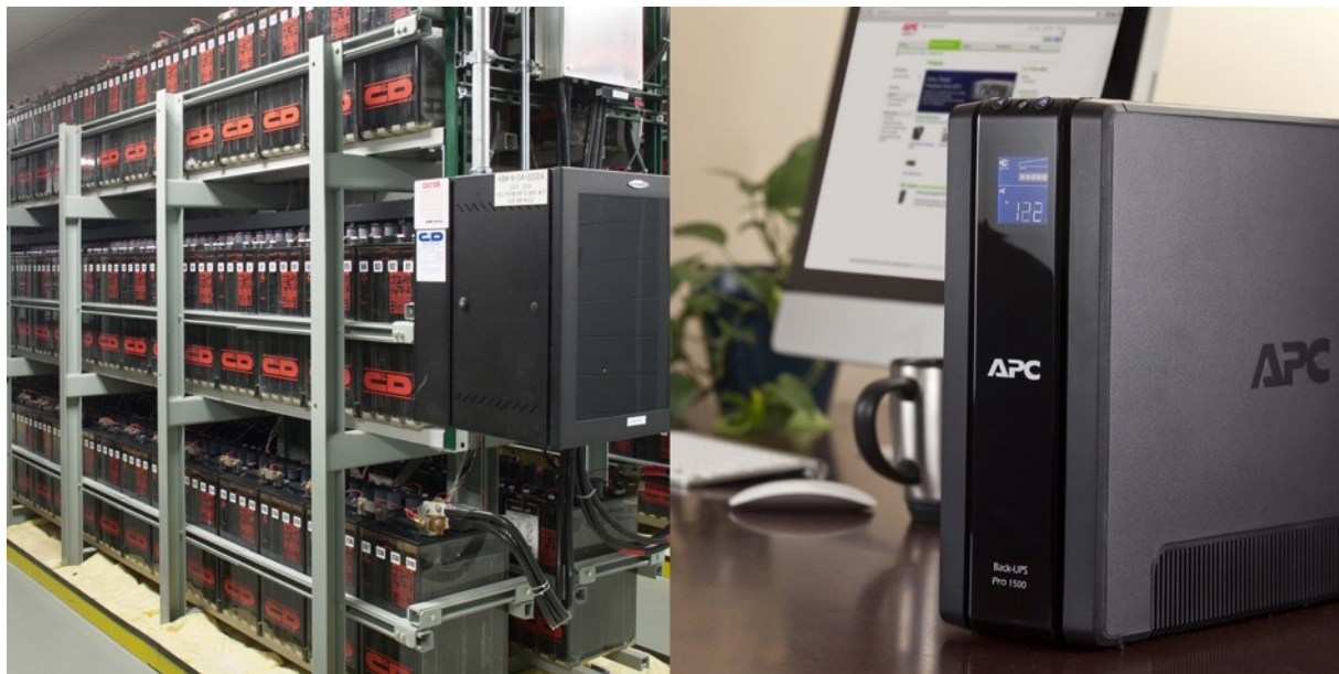
Battery plant and standalone UPS installation
